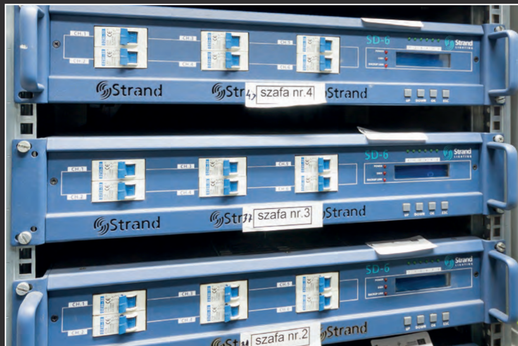
□ REGULATORY NAPIĘCIA SD-6 PHILIPS STRAND LIGHTING
