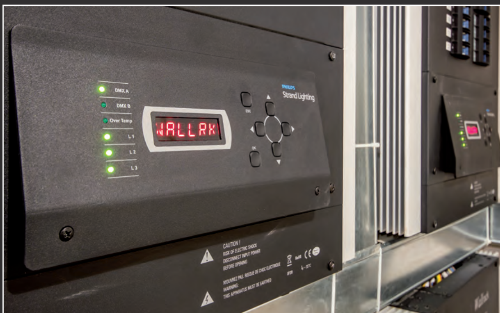
REGULATOR WALLRACK FIRMY PHILIPS STRAND LIGHTING
